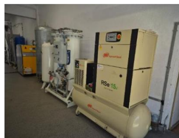
Statia de producer azot
