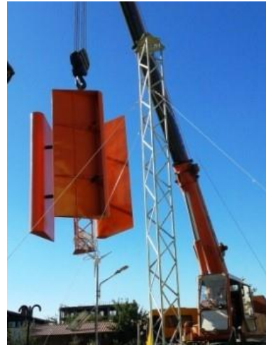
Figure 13. Crane lifting the top of the wind turbine.
