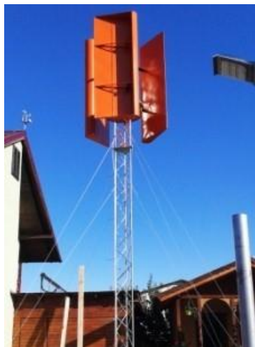
Figure 14. Lenz wind turbine installed.
