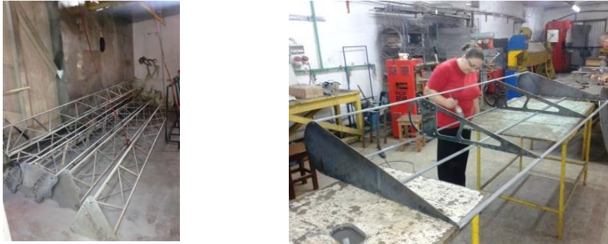
Figure 8. Turbine towers (left) and blade (right) after applying the protective zinc coat.
