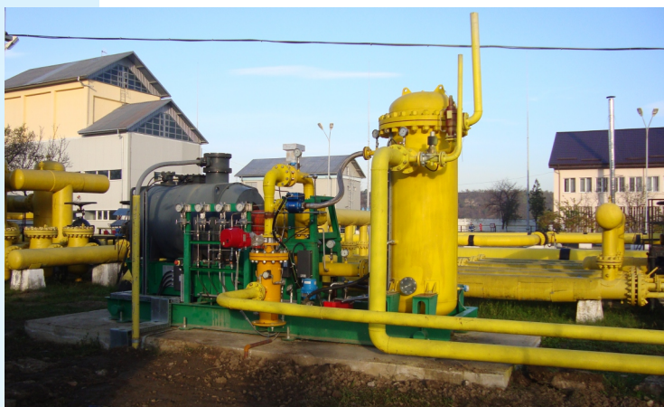
Ansamblu expander elicoidal-generator.
